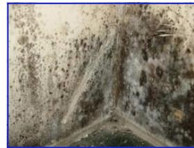
This picture shows the effects of condensation in the corner of a room. Note the way that the black mould climbs and concentrates on the coldest part of the wall – an outside corner
